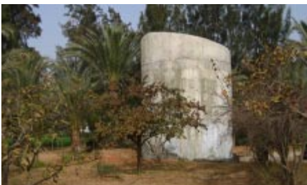
The reservoir shortly before completion
