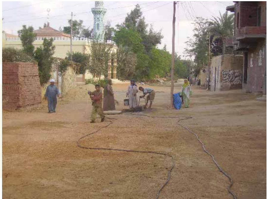
Gelfinas clean streets shine again after extensive cleaning works
